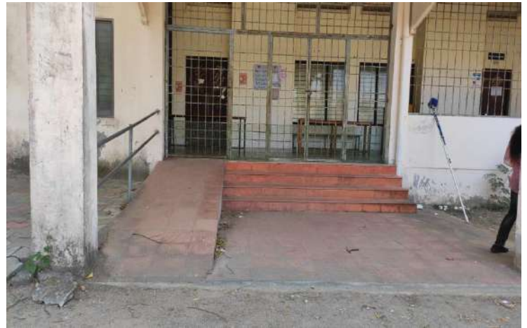
Ramp 2 Main Block
