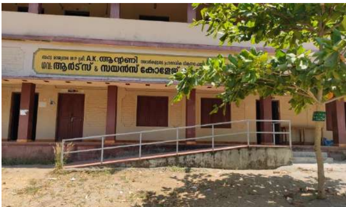
Ramp 1(b) - Microbiology Block
