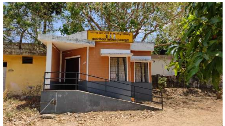
Ramp 3 - Ladies Amenity Centre
