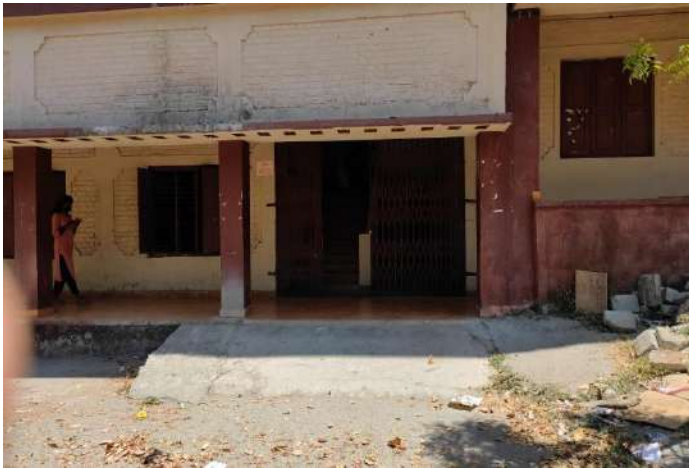
Ramp 1 Microbiology Block
